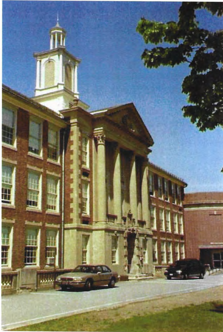
McCall Middle School, Winchester. Photo courtesy of HMFH Architects.
