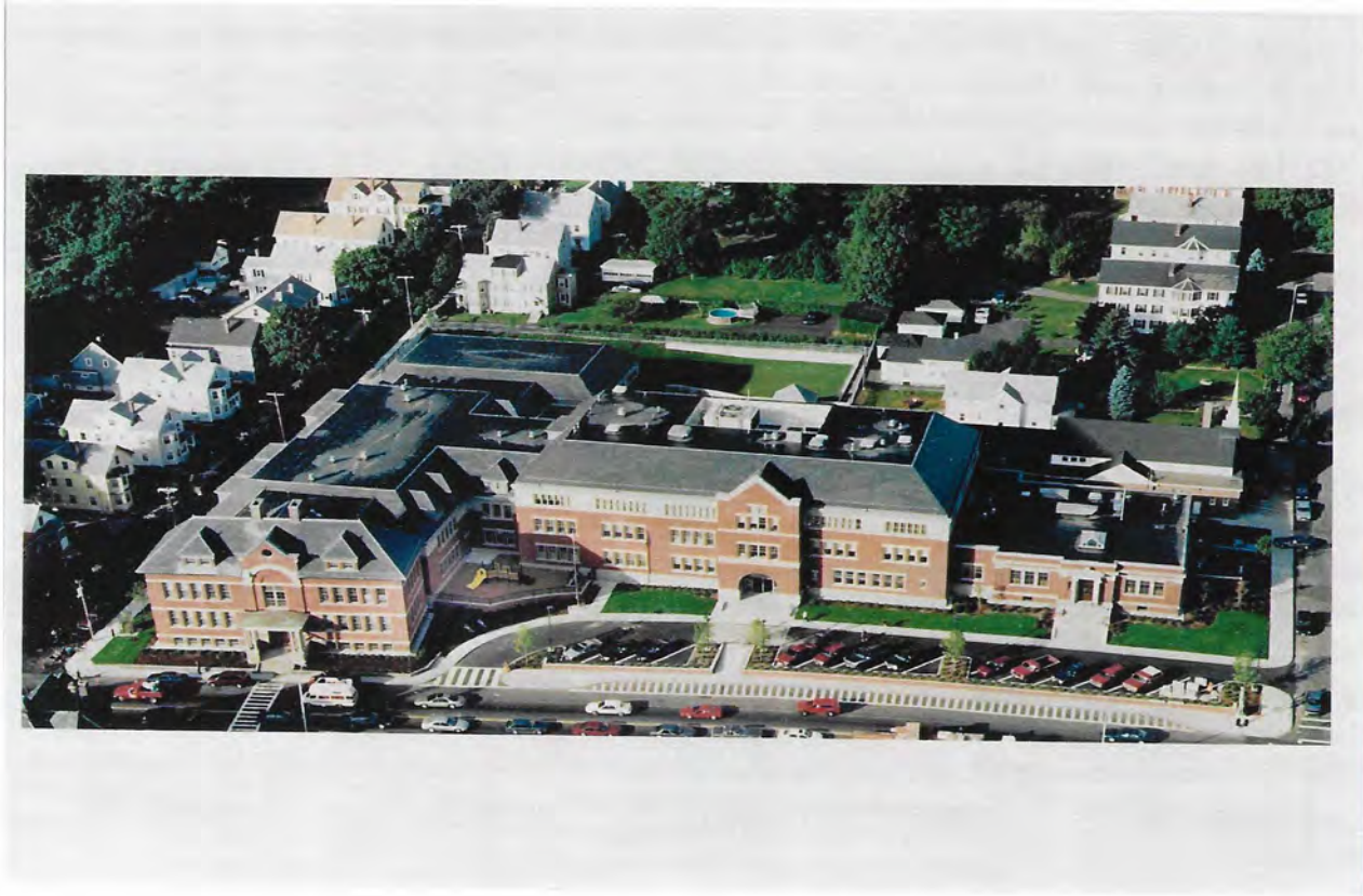
Quinsigamond Elementary School, Worcester. Photo courtesy of Lamoureux*Pagano Associates.
