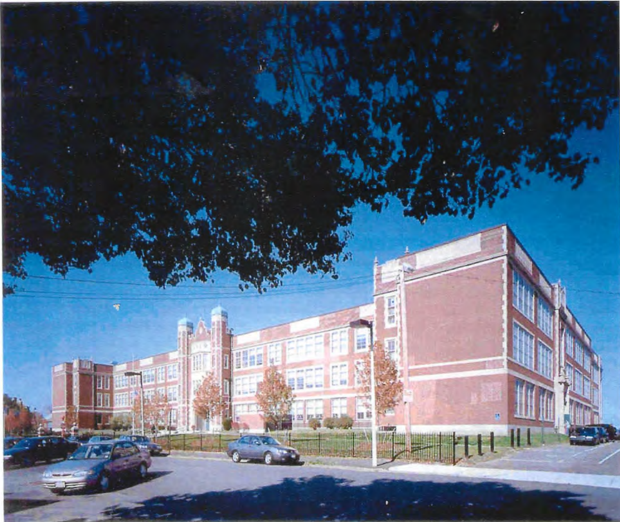
East Boston High School, East Boston. Photo Courtesy of Cole and Goyette, Architects and Planners Inc.
