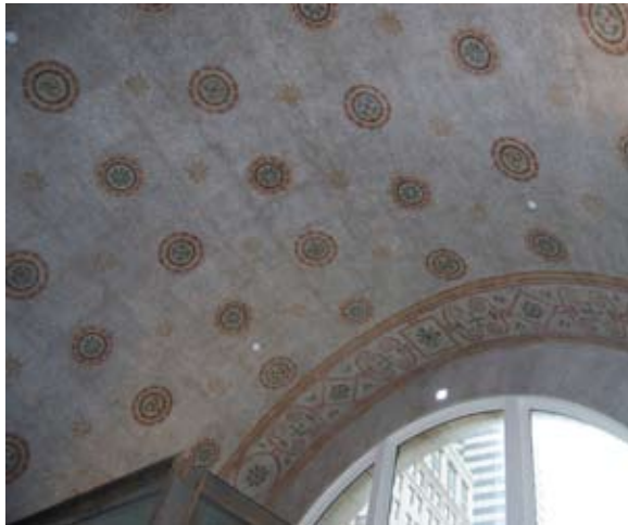
A detailed tile mosaic was preserved on the barrel vaulted ceiling in the main lobby. The Romanesque building is still one of the tallest masonry bearing structures in the United States.
