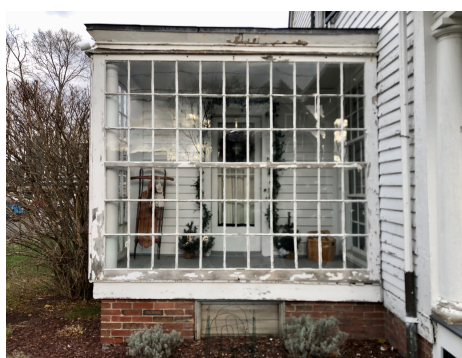
View of windows
