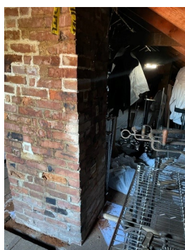
Chimney damage
