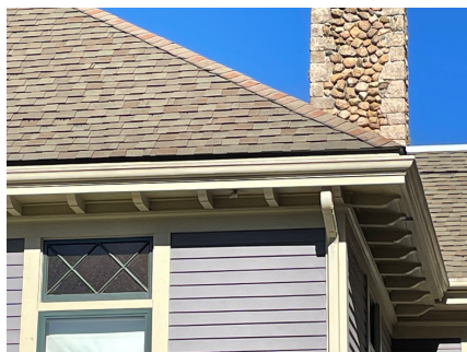
Gutter close up
