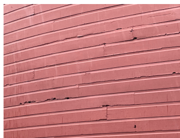
Siding damage
