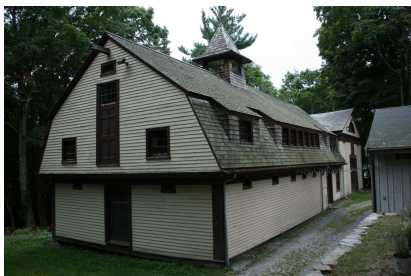
Carriage house view
