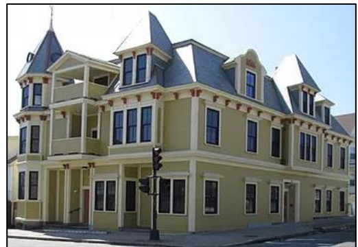
Oscar Romero House after renovations done by Community Action for Better Housing (part of Catholic Social Services), WHALe, and NEI General Contracting.
