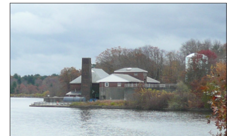
Randolph Water Works, 1889.
