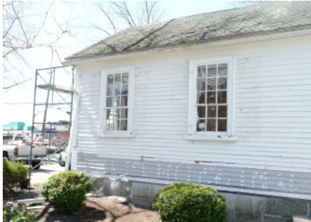
Restoration of 1838 addition to Jonathan Belcher house.
