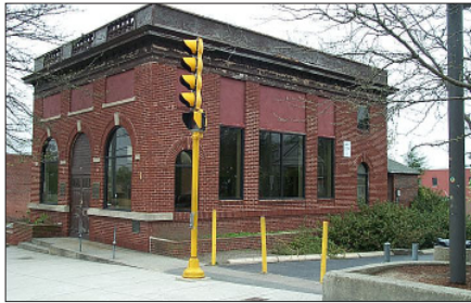
Corkin Building, ca. 1925.
